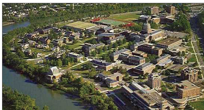
Strong Memorial Hospital and its University at Rochester, NY, USA.
